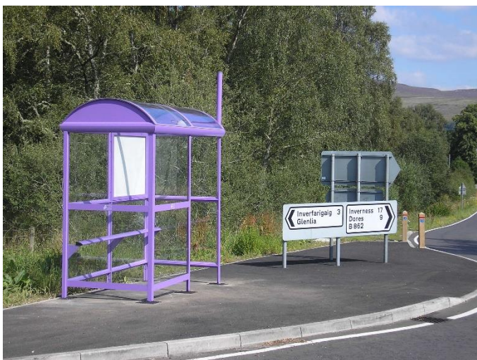
There is a new Bus Shelter at Errogie Corner
