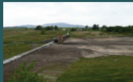
Dam, looking up to the Glebe about 2010 photo thanks to Mr David Johnson
