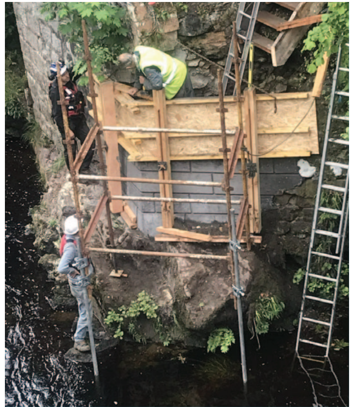
Removing shuttering for 4th concrete pour
